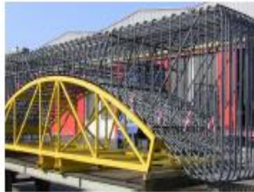
Reinforcement of Concrete Arch Girder
