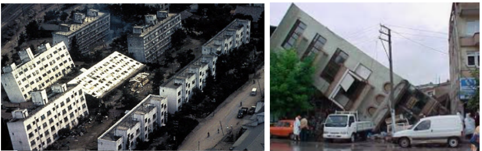
FIGURE 1.5 Building tilt and settlement due to liquefaction during the 1964 Niigata earthquake.
